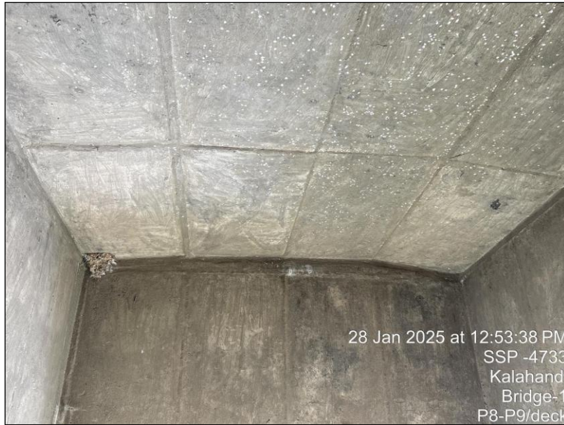
Photo 96: A view of deck slab in the Span P8-P9 of H.L Bridge at 27/500 Km on Bhawanipatna-Khariar Road in the Kalahandi Division.
