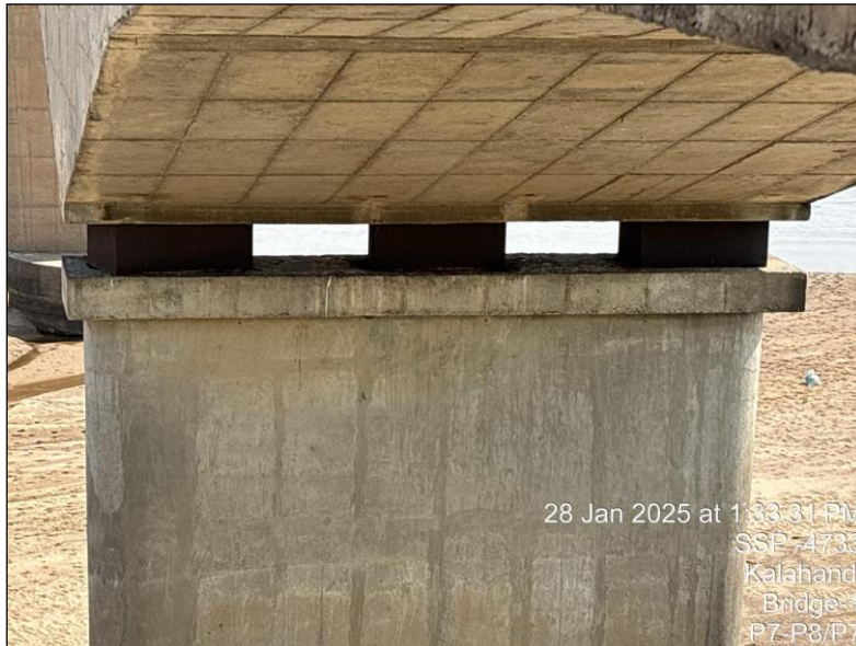
Photo 50: A view of Roller-cum-Rocker bearing at Pier P-7 in the Span P7-P8 of H.L Bridge at 27/500 Km on Bhawanipatna-Khariar Road in the Kalahandi Division.
