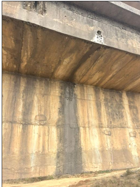
Photo 189: A typical view of drainage spout of H.L Bridge at 27/500 Km on Bhawanipatna-Khariar Road in the Kalahandi Division
