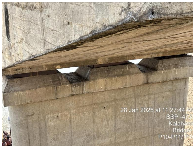
Photo 131: A view of Pier P-10 in the Span P10-P11 of H.L Bridge at 27/500 Km on Bhawanipatna-Khariar Road in the Kalahandi Division
