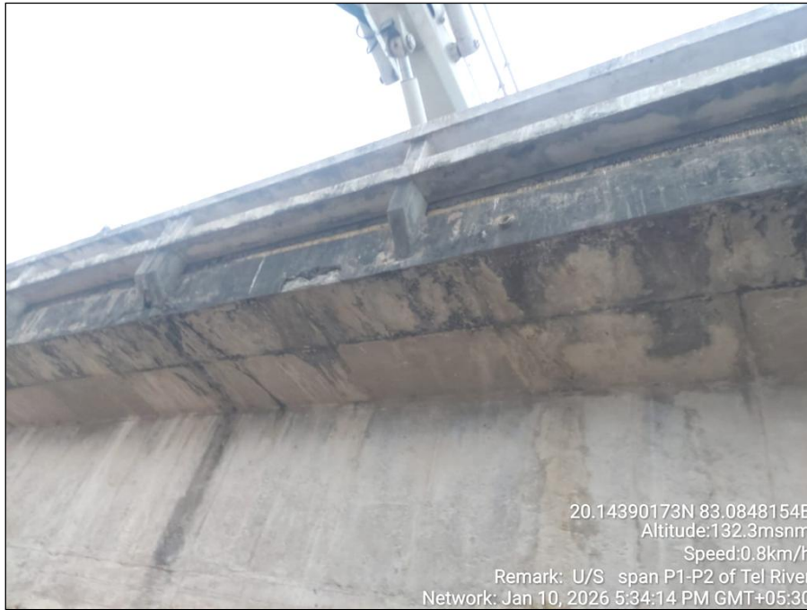
Photo 159: A view of side drains on u/s web of distressed Span P11-P12 of H.L Bridge at 27/500 Km on Bhawanipatna-Khariar Road in the Kalahandi Division
