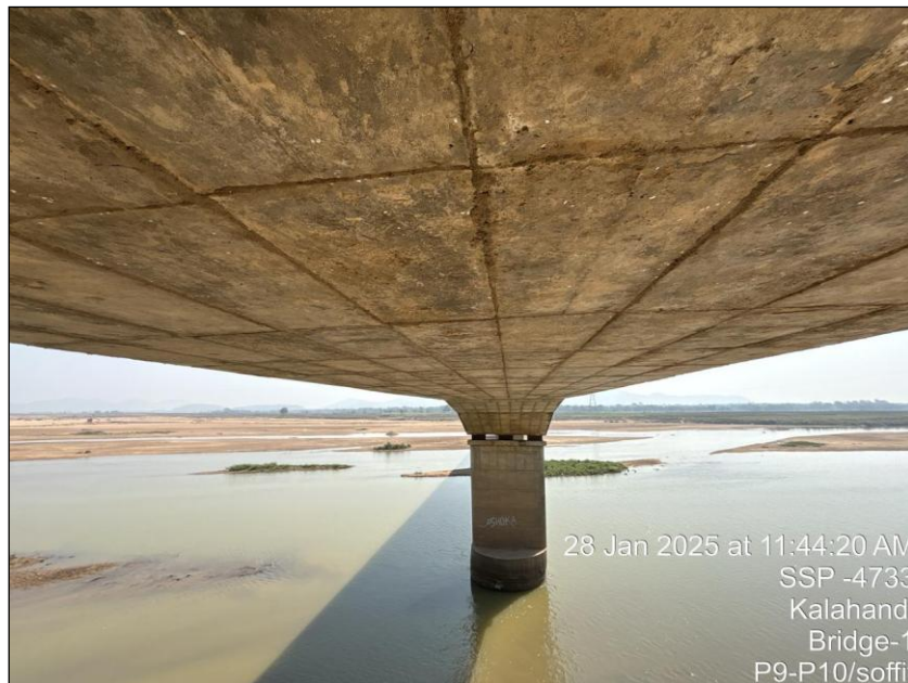
Photo 109: A view of Pier P-9 in the Span P9-P10 of H.L Bridge at 27/500 Km on Bhawanipatna-Khariar Road in the Kalahandi Division
