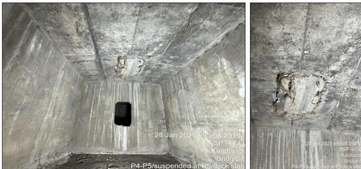
Photo 19: A view of repaired shear punching on the deck slab near pier P-5 in the Span P4-P5 of H.L Bridge at 27/500 Km on Bhawanipatna – Khariar Road in the Kalahandi Division.
