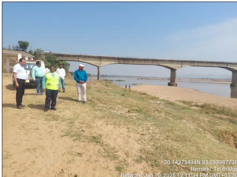
Photo 164: A view of Joint Inspection of H.L Bridge at 27/500 Km on Bhawanipatna-Khariar Road in the Kalahandi Division
