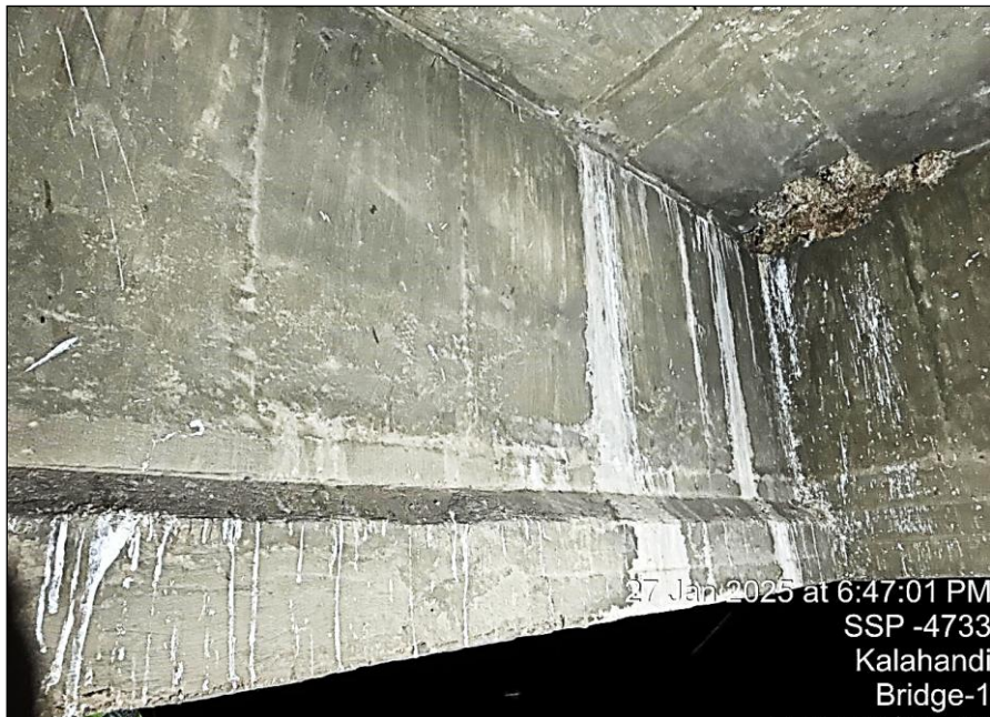
Photo 128: A view of girder G2 in the Span P10-P11 of H.L Bridge at 27/500 Km on Bhawanipatna-Khariar Road in the Kalahandi Division.
