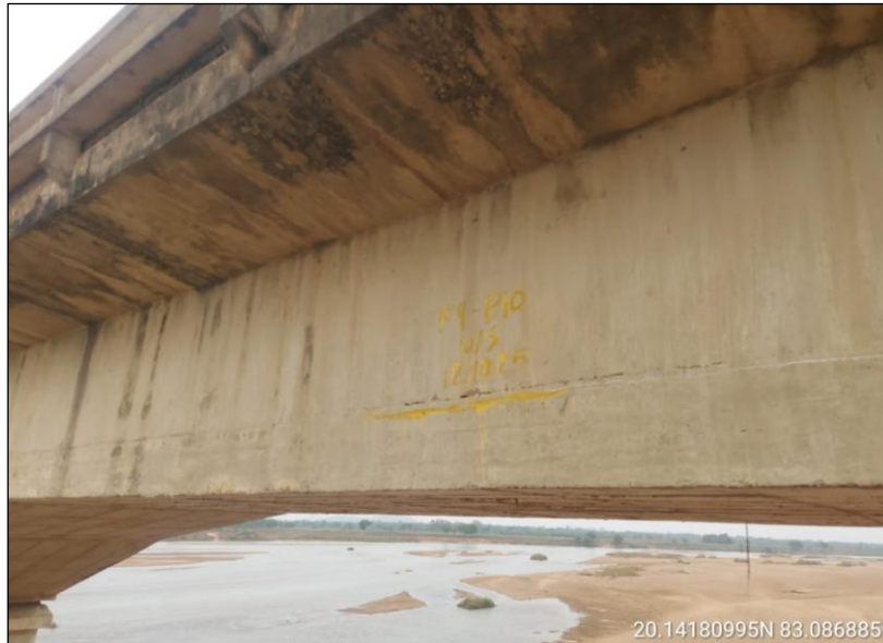
Photo 16: A view of the Web (u/s) in the Span P3-P4 of H.L Bridge at 27/500 Km on Bhawanipatna–Khariar Road in the Kalahandi Division.
