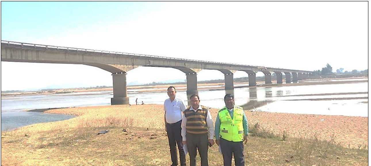
Photo 2(a): A U/S view of H.L Bridge at 27/500 Km on Bhawanipatna - Khariar Road in the Kalahandi Division.
