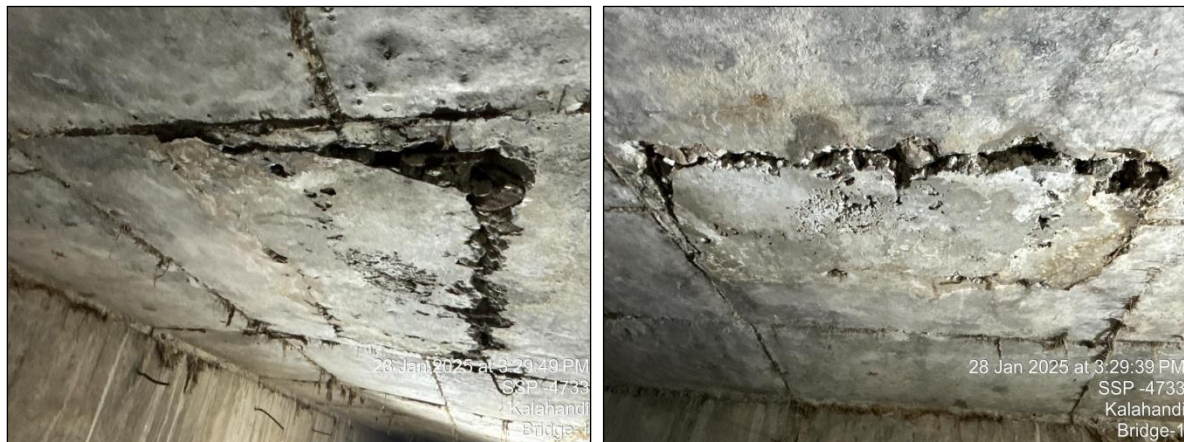
Photo 77: A view of repaired shear punching patch work on Deck Slab in cell-2 near Pier P-7 In the suspended Span P7-P8 of H L Bridge at 27/500 Km on Bhawanipatna-Khariar Road in the Kalahandi Division
