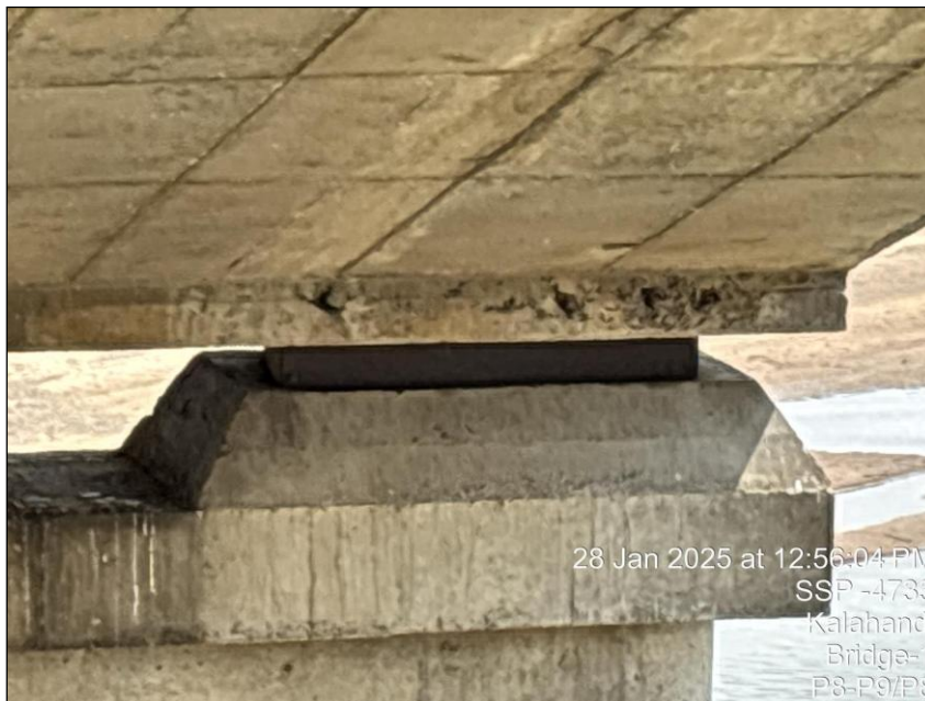
Photo 87: A view of bearing at Pier P-8 in the Span P8-P9 of H L Bridge at 27/500 Km on Bhawanipatna-Khariar Road in the Kalahandi Division.
