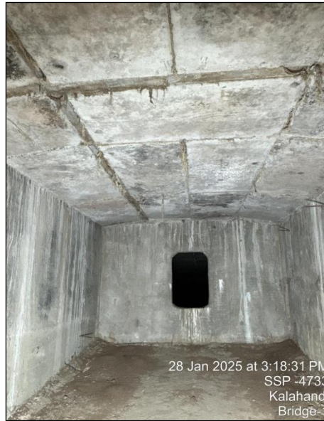
Photo 66: A view of Deck Slab in Cell-1 near pier P-7 in the Span P7-P8 of H L Bridge at 27/500 Km on Bhawanipatna-Khariar Road in the Kalahandi Division.
