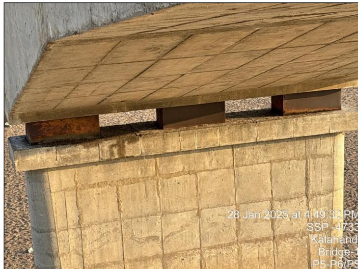
Photo 20: A view of Cut-Roller-cum-Rocker bearing on Pier P-5 in the Span P5-P6 of H.L Bridge at 27/500 Km on Bhawanipatna – Khariar Road in the Kalahandi Division
