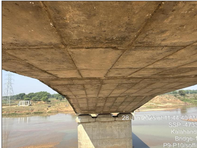
Photo 110: A view of bottom surface near Pier P-10 in the Span P9-P10 of H.L Bridge at 27/500 Km on Bhawanipatna-Khariar Road in the Kalahandi Division
