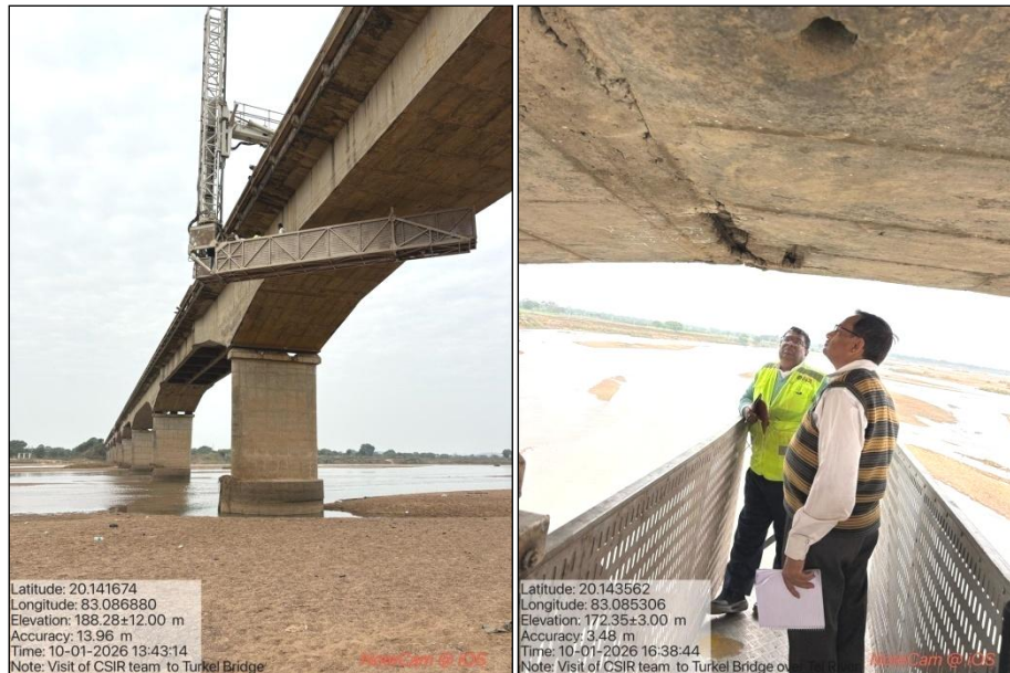
Photo 2(c): A view Inspection of distressed H.L Tel Bridge at 27/500 Km on Bhawanipatna - Khariar Road in the Kalahandi Division.
