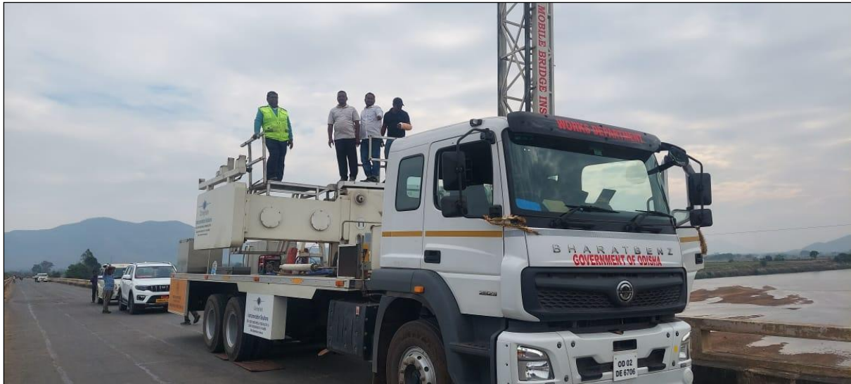
Photo 2(b): A U/S view of H.L Bridge at 27/500 Km on Bhawanipatna - Khariar Road in the Kalahandi Division.
