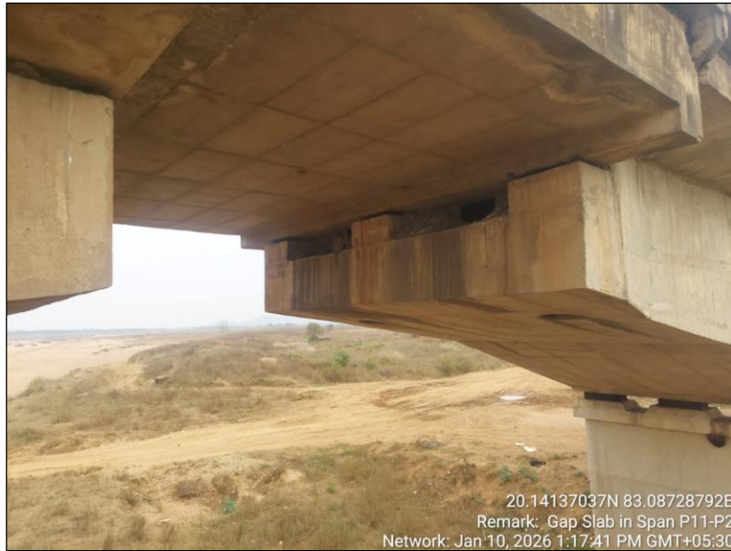
Photo 12(a):A view of Gap Slab in the span P1-P2 of Tel Bridge of the Kalahandi Section.
