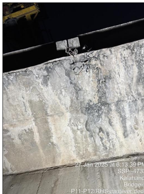
Photo 160: A view of RHS Cantilever Deck Slab in the Span P11-P12 of H.L Bridge at 27/500 Km on Bhawanipatna-Khariar Road in the Kalahandi Division
