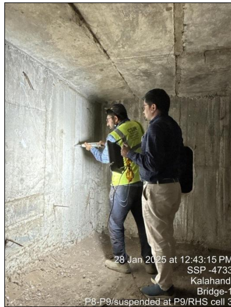
Photo 98: A view of Rebound hammer test on RHS web wall in cell-3 (longitudinal) at pier P-9 in the Span P8-P9 of H L Bridge at 27/500 Km on Bhawanipatna-Khariar Road in the Kalahandi Division
