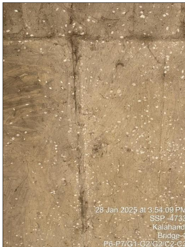
Photo 37: A view of Deck Slab Between girder G1-G2 and Cross girder C2-C3 of H.L Bridge at 27/500 Km on Bhawanipatna–Khariar Road in the Kalahandi Division.
