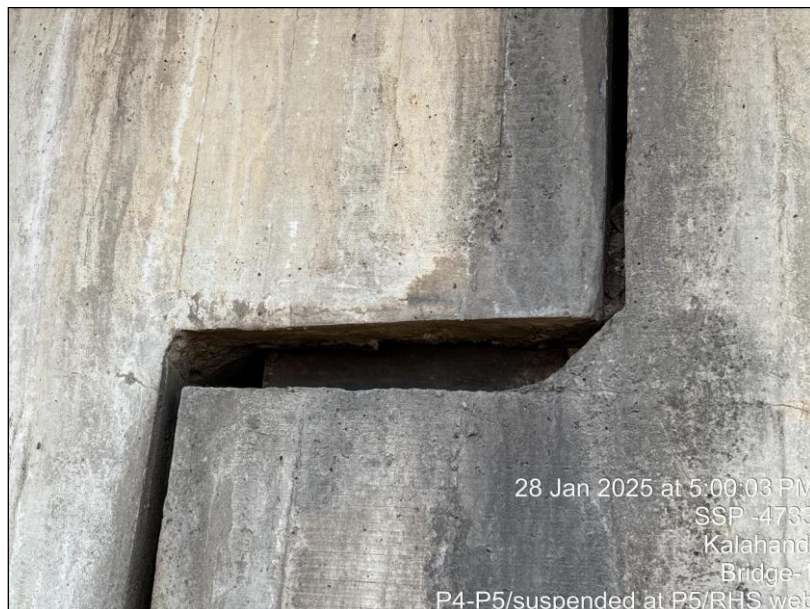
Photo 17: A view of Rocker bearing in suspended Span P4-P5 of H.L Bridge at 27/500 Km on Bhawanipatna–Khariar Road in the Kalahandi Division
