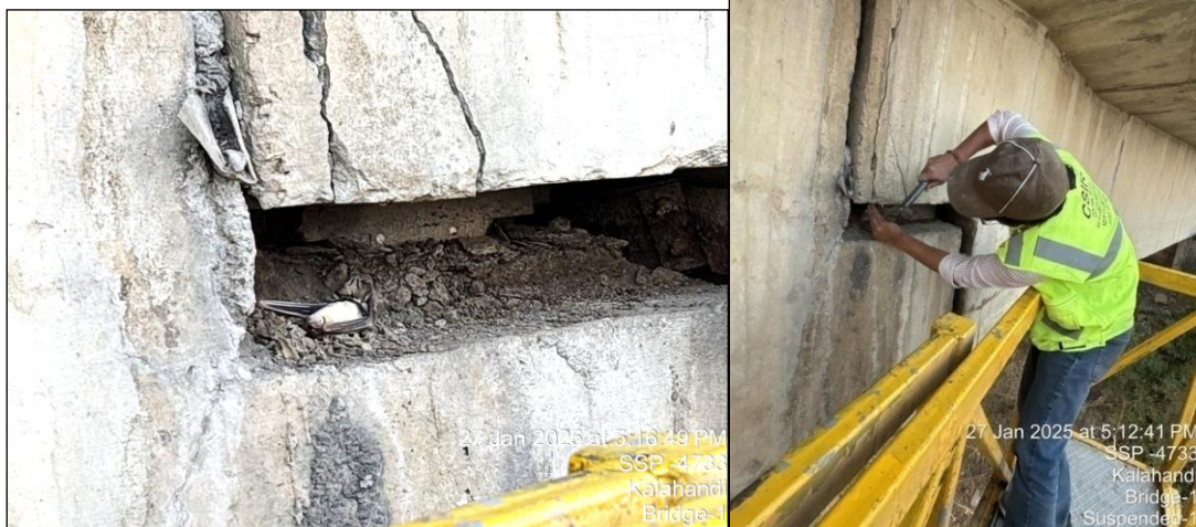
Photo 170: A view of Rocker Bearing in the Span P12-A2 of H.L Bridge at 27/500 Km on Bhawanipatna – Khariar Road in the Kalahandi Division.
