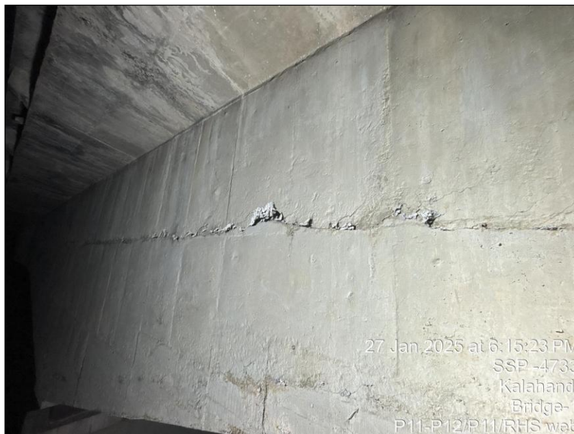
Photo 147: A view of construction joint on the RHS web in the span P11-P12 of H.L Bridge at 27/500 Km on Bhawanipatna-Khariar Road in the Kalahandi Division.
