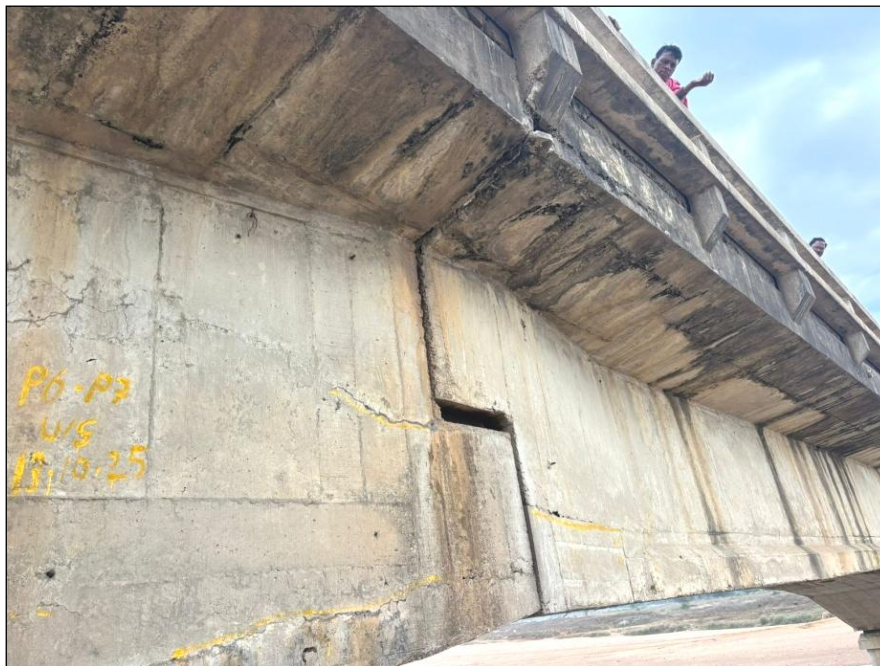
Photo 39: A view of Span P6-P7 of HL Bridge at 27/500 Km on Bhawanipatna–Khariar Road in the Kalahandi Division.
