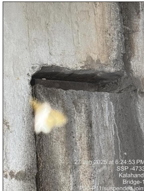
Photo 134: A view of Rocker Bearing on Suspended Span P10-P11 of H.L Bridge at 27/500 Km on Bhawanipatna-Khariar Road in the Kalahandi Division
