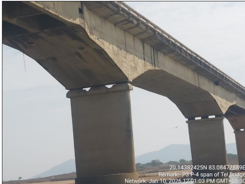
Photo 102: A view of Span P9-P10 of H.L Bridge at 27/500 Km on Bhawanipatna-Khariar Road in the Kalahandi Division.
