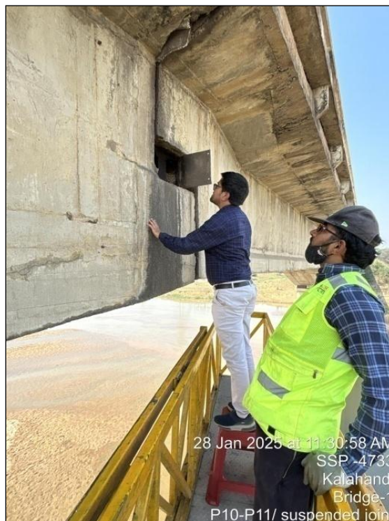
Photo 123: A view of Inspection of Roller bearing of Suspended span in the span P10-P11 of H.L Bridge at 27/500 Km on Bhawanipatna-Khariar Road in the Kalahandi Division
