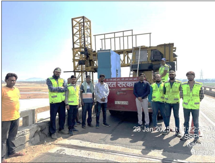
Photo 3: A view of joint Inspection through MBIU of H.L Tel Bridge at 27/500 Km on Bhawanipatna–Khariar Road in the Kalahandi Division.
