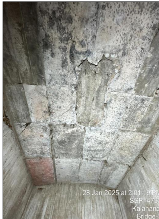
Photo 82: A view of repaired patch work on Deck Slab near Pier P-7 in the Span P7-P8 of H.L Bridge at Km 27/500 Km on Bhawanipatna-Khariar Road in the Kalahandi Division.
