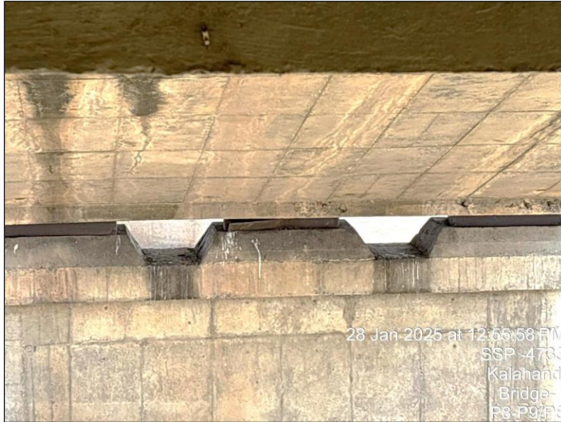
Photo 86: A view of bearing at Pier P-8 in the Span P8-P9 of H.L Bridge at 27/500 Km on Bhawanipatna-Khariar Road in the Kalahandi Division
