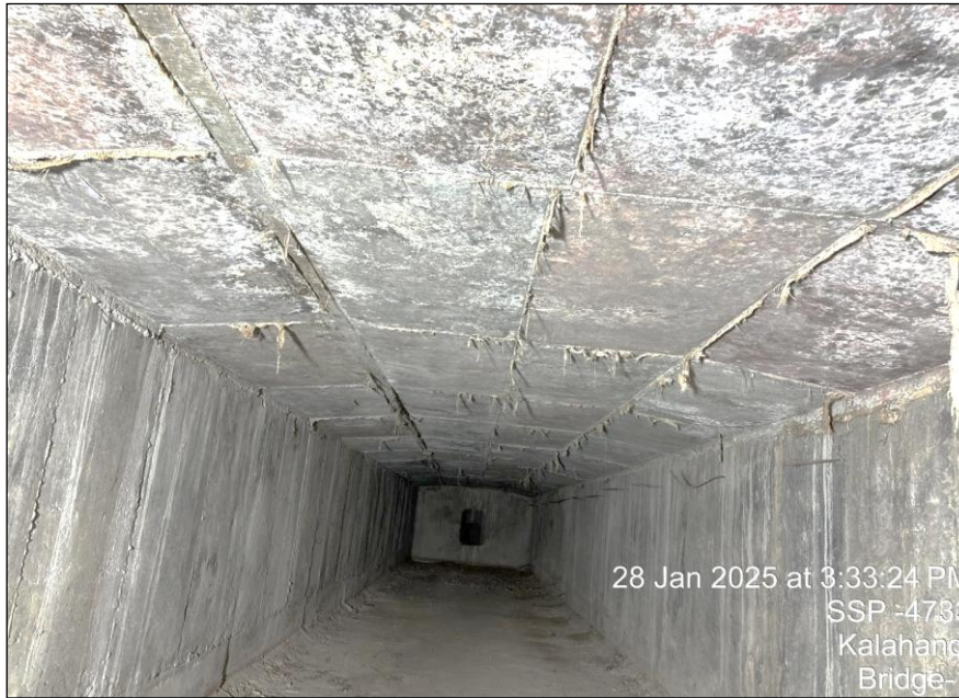
Photo 72: A view of deck slab in Cell-2 near Pier P-7 in the Suspended Span P7-P8 of HL Bridge at 27/500 Km on Bhawanipatna-Khariar Road in the Kalahandi Division.
