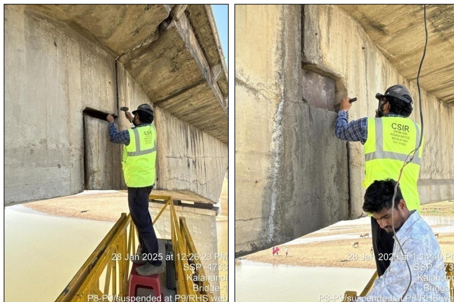
Photo 99: A view of inspection of bearings in the Span P8-P9 of H L Bridge at 27/500 Km on Bhawanipatna-Khariar Road in the Kalahandi Division.
