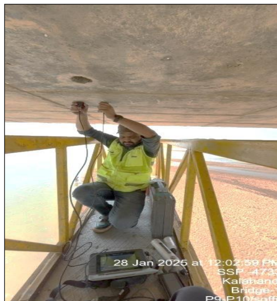
Photo 115: A view of UPV test on Soffit slab in the span P9-P10 of H.L Bridge at 27/500 Km on Bhawanipatna-Khariar Road in the Kalahandi Division
