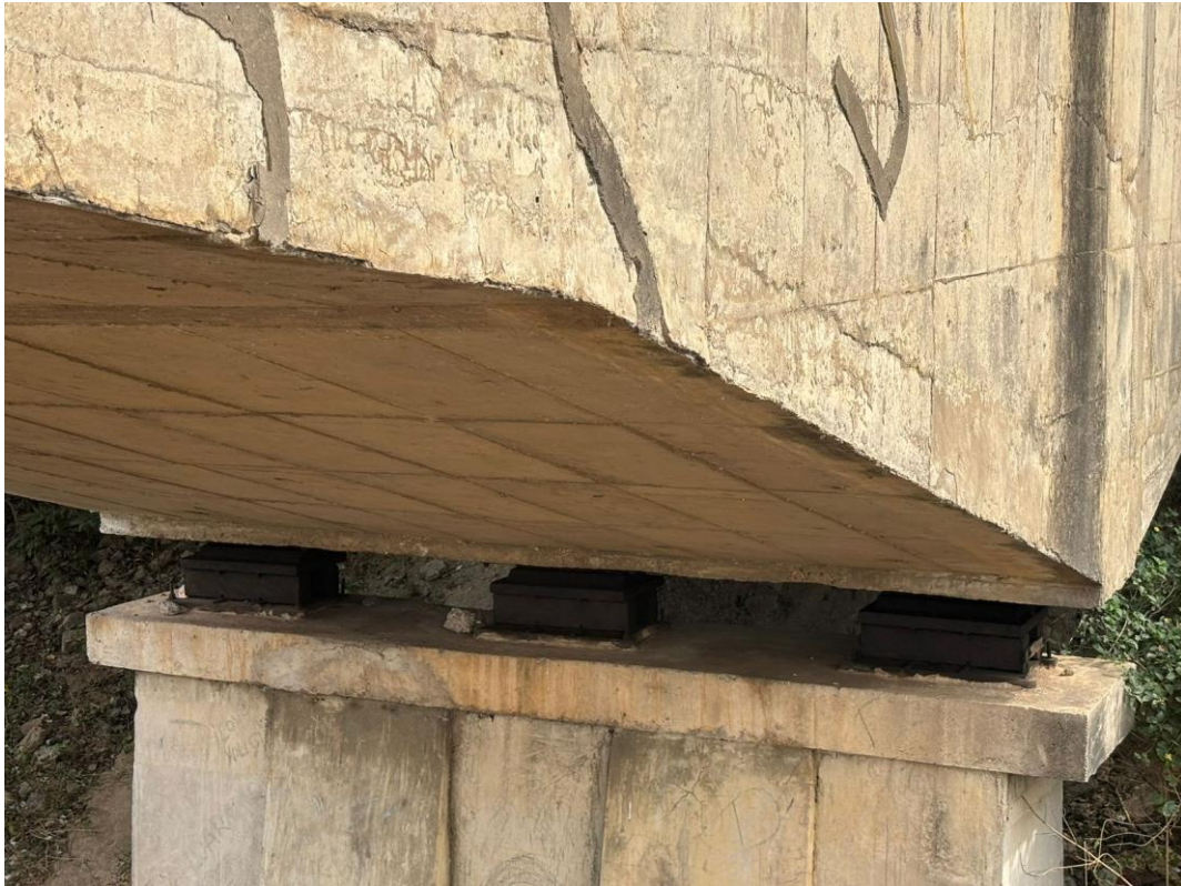
Photo 9(b): A view of Rocker-cum-cut Roller bearings at Abutment A-1 of the H.L Tel Bridge at 27/500 Km on Bhawanipatna–Khariar Road in the Kalahandi Division
