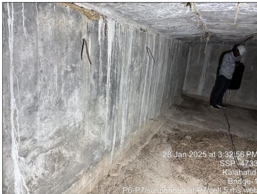
Photo 75: A view of RHS web in Cell-2 near Pier P-7 in the Span P7-P8 of H.L Bridge at 27/500 Km on Bhawanipatna-Khariar Road in the Kalahandi Division
