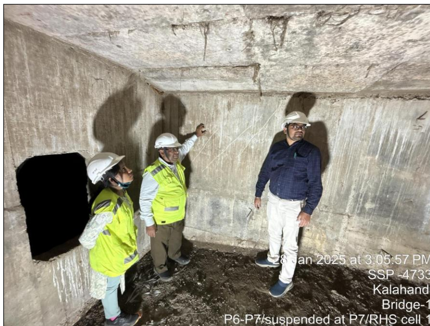
Photo 41: A view of inspection inside RHS cell-1 near Pier P-7 of Box girder in the Suspended Span P6-P7 of HL Bridge at 27/500 Km on Bhawanipatna–Khariar Road in the Kalahandi Division.
